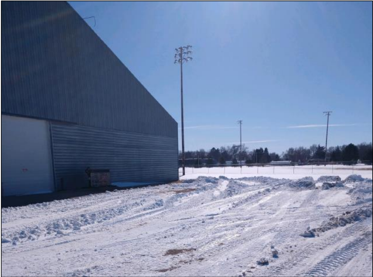
Photo of Plowed Area in Front of S.O.S. Storage Building
