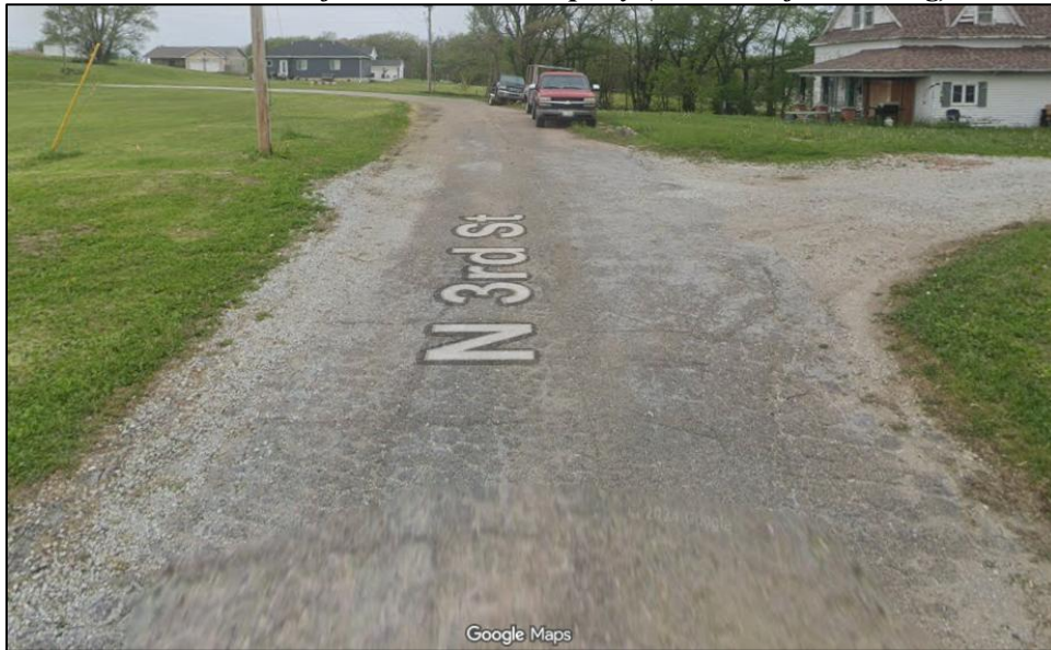
Road in Front of Mr. Weible's Property (2023 – Before Paving)
