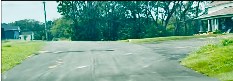
Road in Front of Mr. Weible's Property (2025 – After Paving)
