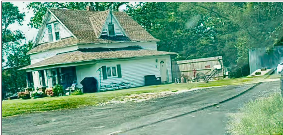
Connecting Road Next to Mr. Weible's Property (2025 – After Paving)
